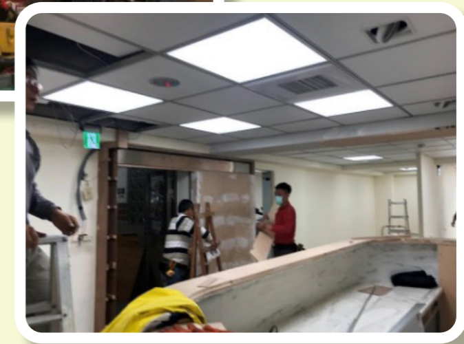
▲ Replacement of old air conditioners and lamps with inverter air conditioners and LED lamps at our Tainan office.
